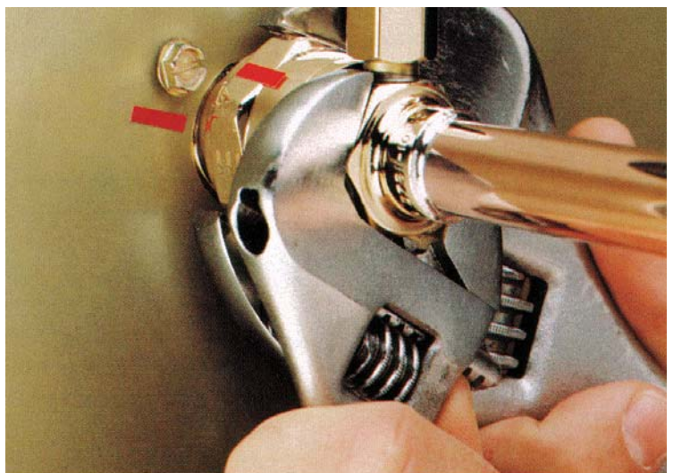
Rotate Each Swivel Nut \frac{1}{4} Turn More
