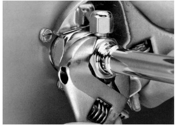
Tighten Swivel Nut
