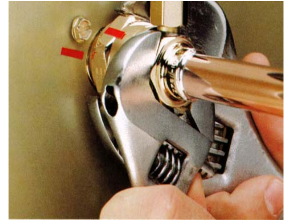
Rotate Swivel Nut One Quarter Turn More After Nut Becomes Tight
