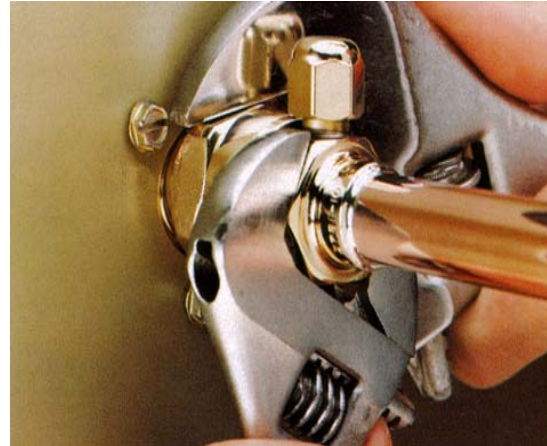
Use Two Wrenches to Tighten
